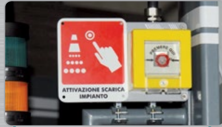
Fire extinguish system
